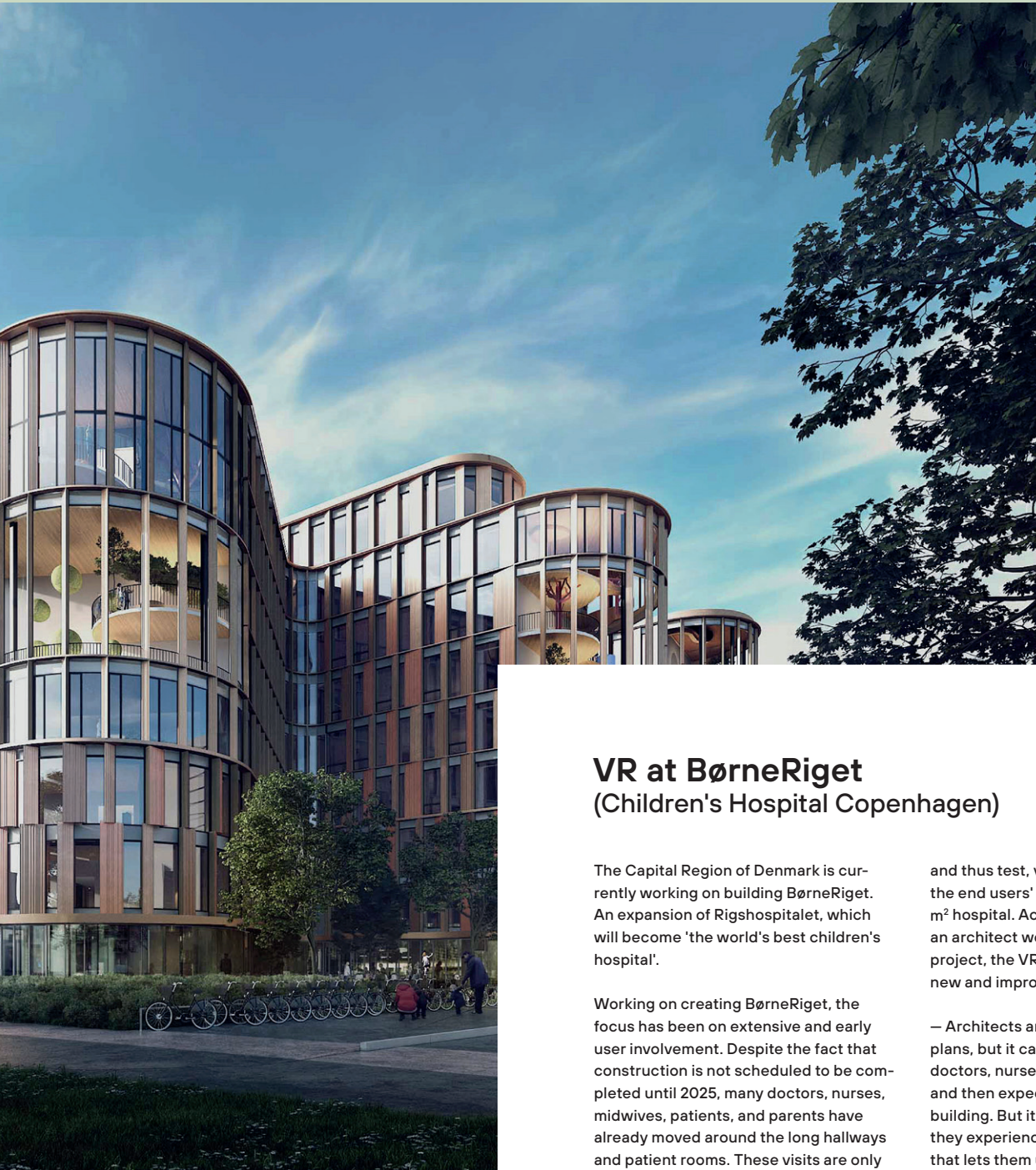
BørneRiget (Children's Hospital Copenhagen) is scheduled to be completed in 2025. Illustration: 3XN
